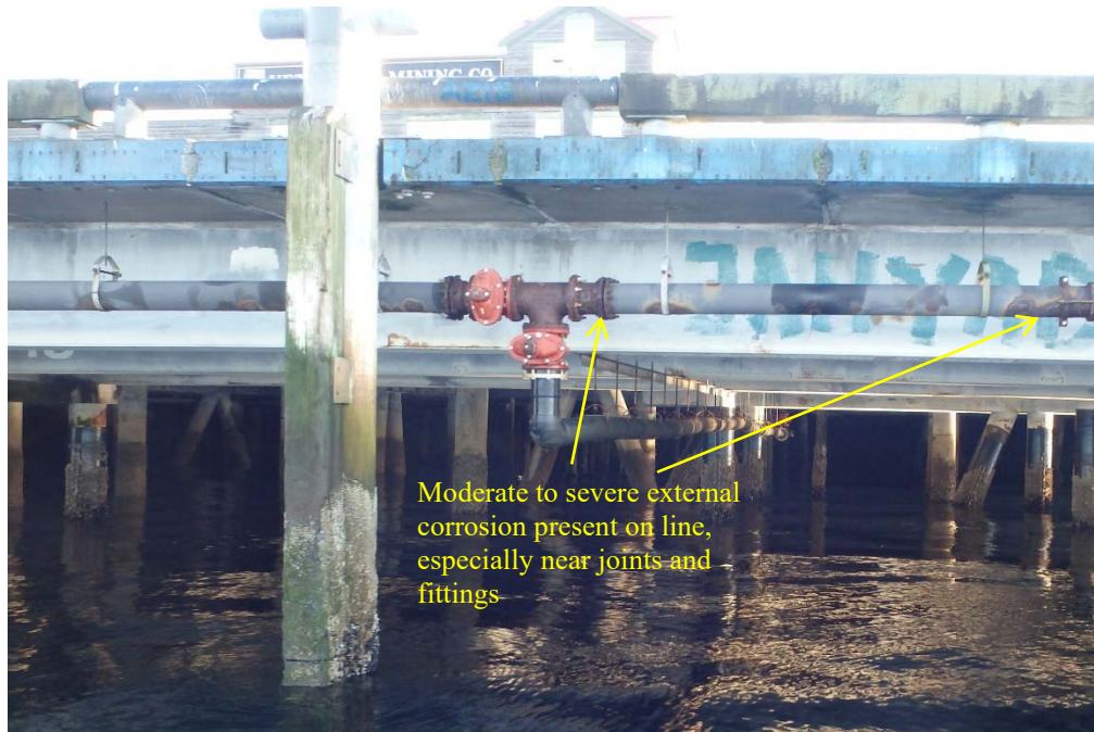
Figure 8: Water line (6") and hanger supports beneath berth
