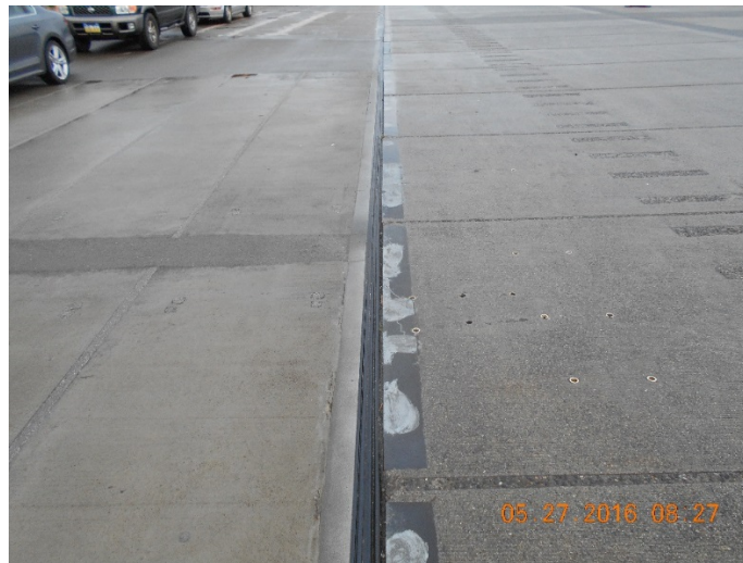
Figure 33: Expansion Joint
