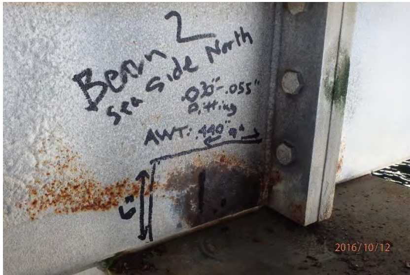
Beam 2, sea side, north of flange (UT Location 2)
