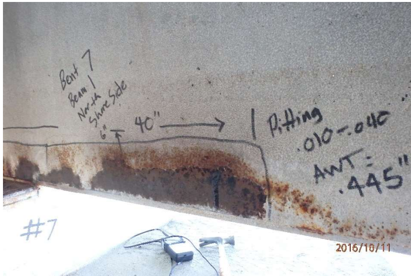
Beam 1, shore side, north of piling cap (UT Location 2)
