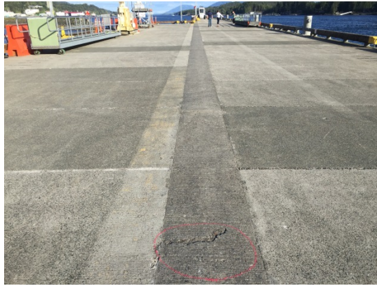
Figure 6: Panel End Joints at Box Girder
