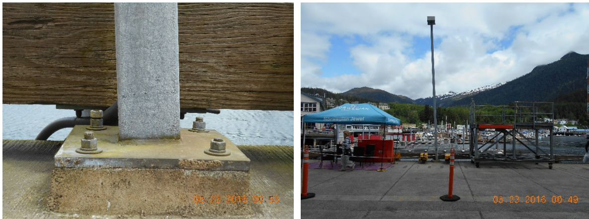
Figure 47: Damaged Light Pole Bases
