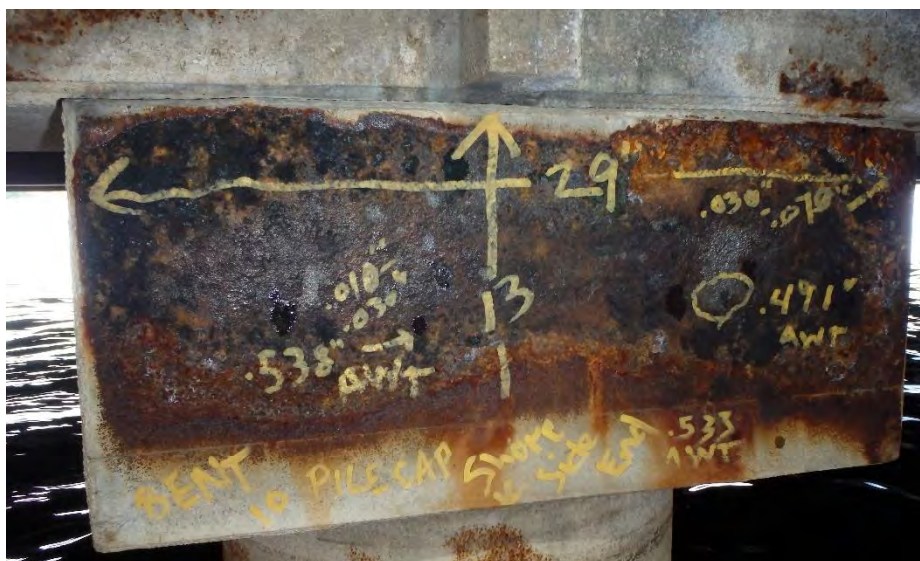
Piling cap sea side end plate (UT Location 2)
