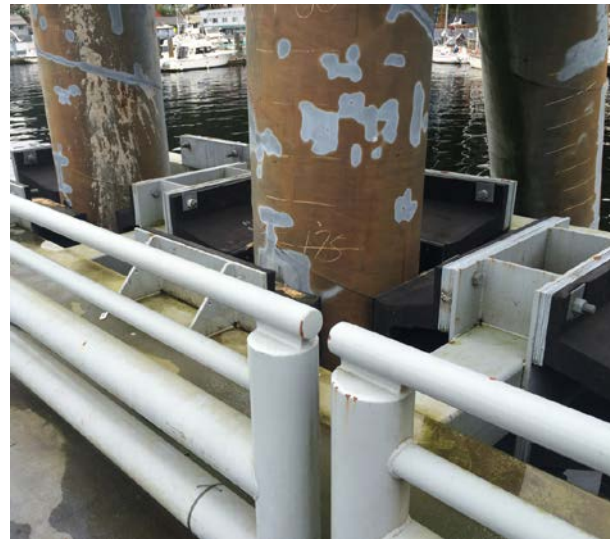
Figure 19: Guide Piling
