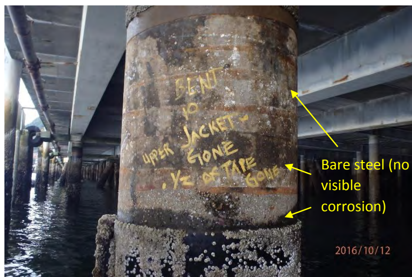
Piling with missing or slipped upper jacket
