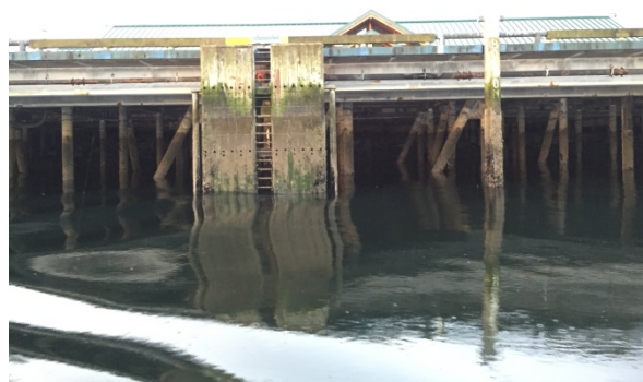
Figure 37: Fender Panel with Bound Fender (submerged)
