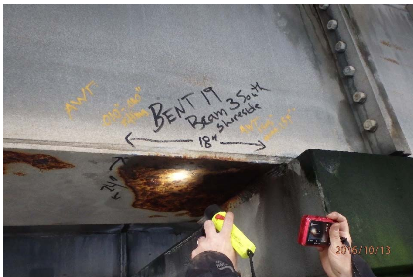
Beam 3 exam area marked with UT and pitting notes
