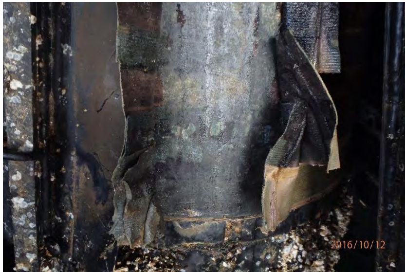
As-found condition of piling steel surface (no visible corrosion)
