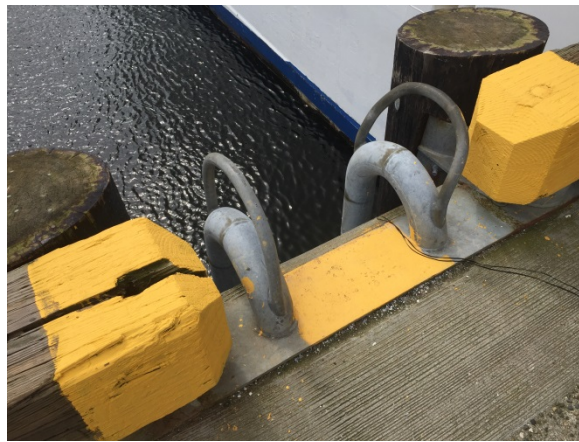
Figure 46: Bent Ladder Rail
