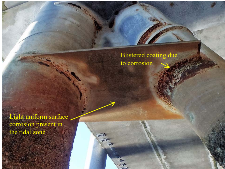
Figure 17: Berth 3 typical pile surfaces with uniform surface corrosion and coating blistering
