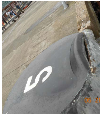
Figure 39: Damaged Bollard Cap
