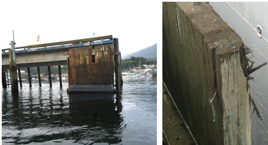
Figure 38: damaged Fender Planks
