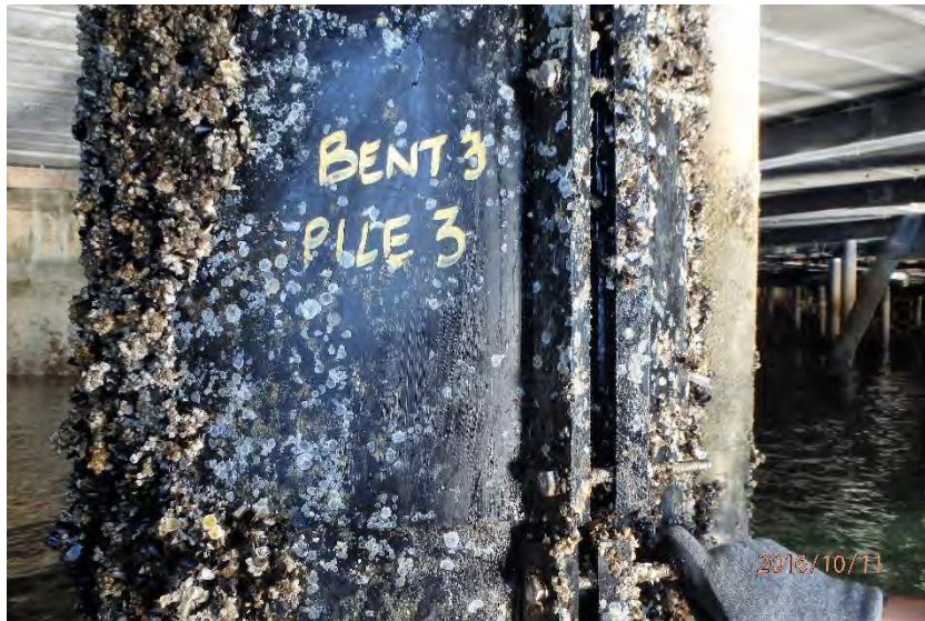
Bent 3 Pile 3 jacket, before opening for examination
