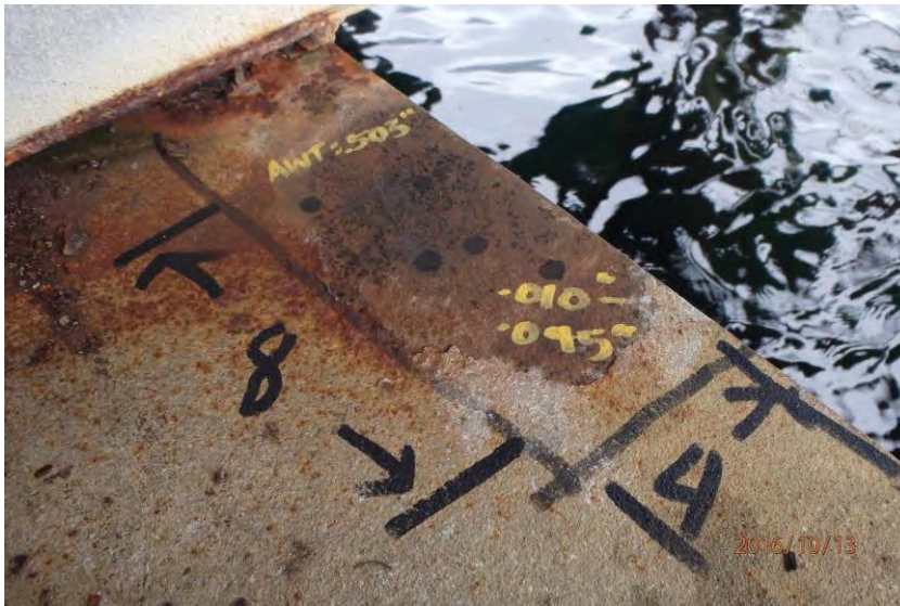
piling cap (UT Location 2)
