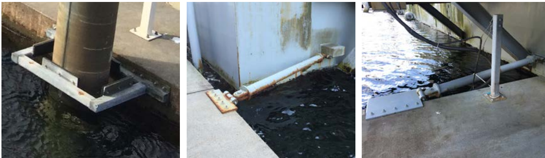
Figure 29b: Guide Piles, Pipe Struts
