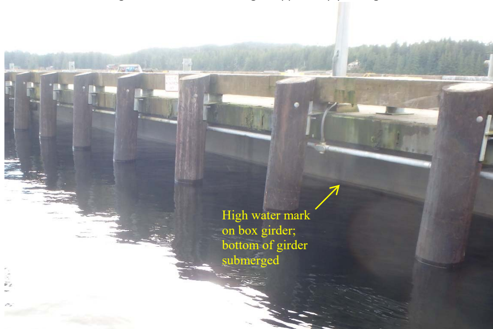
Figure 12: High water mark on box girder (Taken 12:18 on 10/14/16, high tide 16.7 ft)
