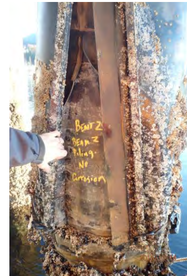
Pile sleeve, no corrosion
