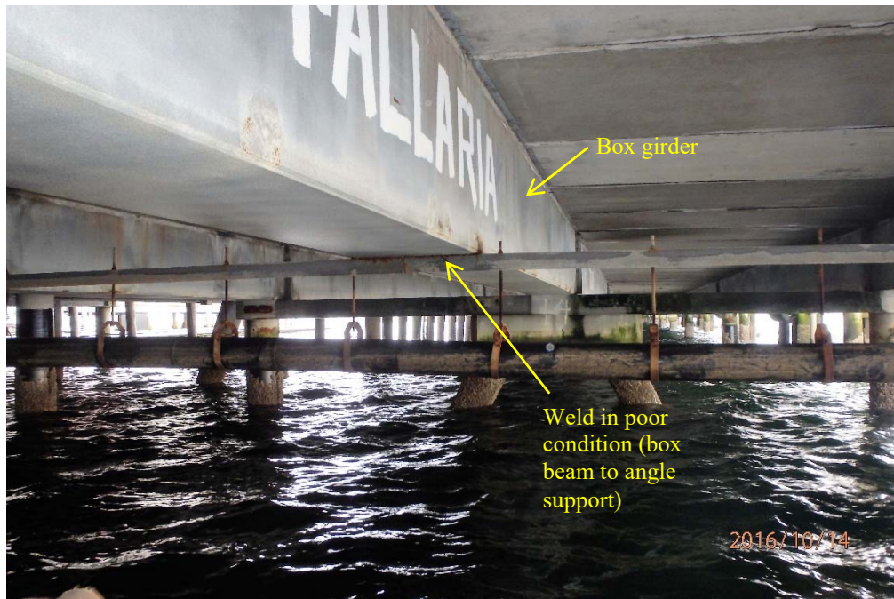
Figure 9: Water line hanger running east/west between Bents 13 and 14
