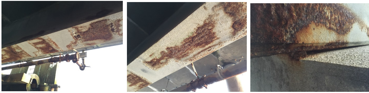
Figure 34: Box Girder Corrosion
