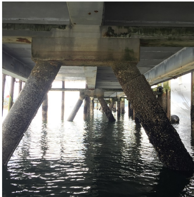
Figure 35: Pile Cap and Sub Cap Corrosion
