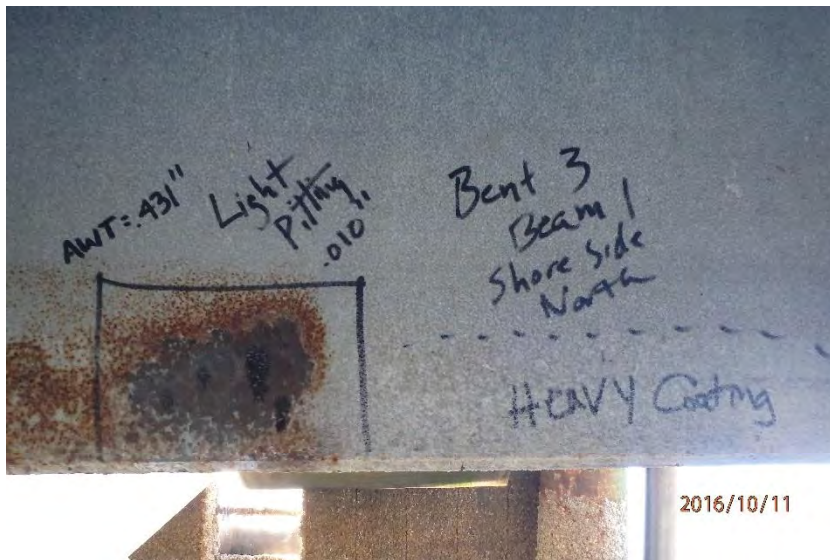
Beam 1 shore side, north end (UT Location 2)
