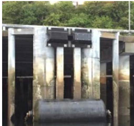
Figure 54: Fender Missing UHMW-PE
