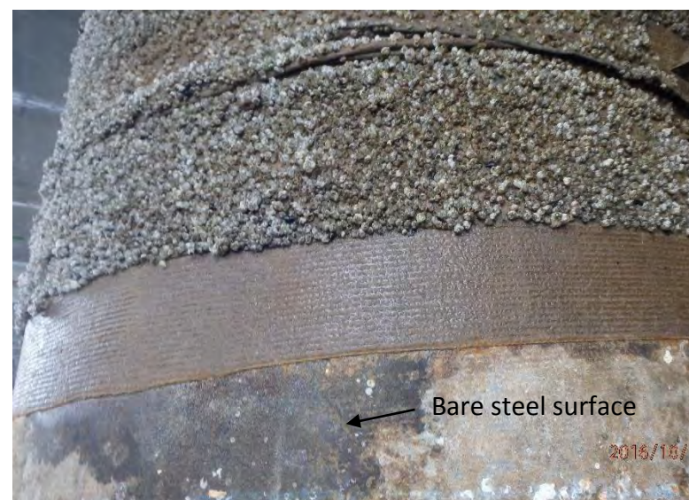
Close-up of piling exposed steel surface
