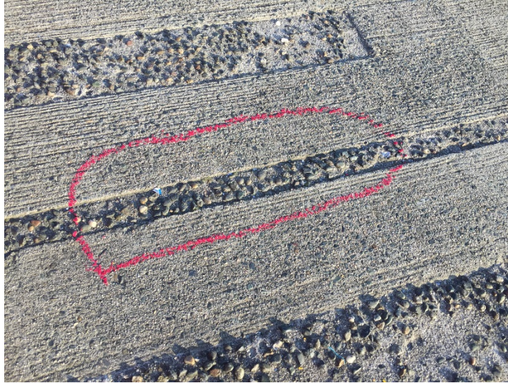
Figure 31: Apparent Grout Voids
