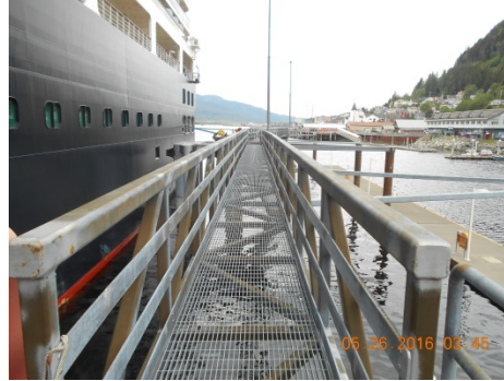
Figure 55: Catwalk Corrosion
