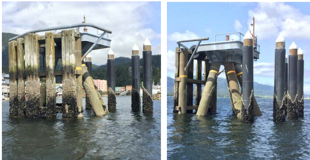
Figure 40: Damaged Bullrail Sections
