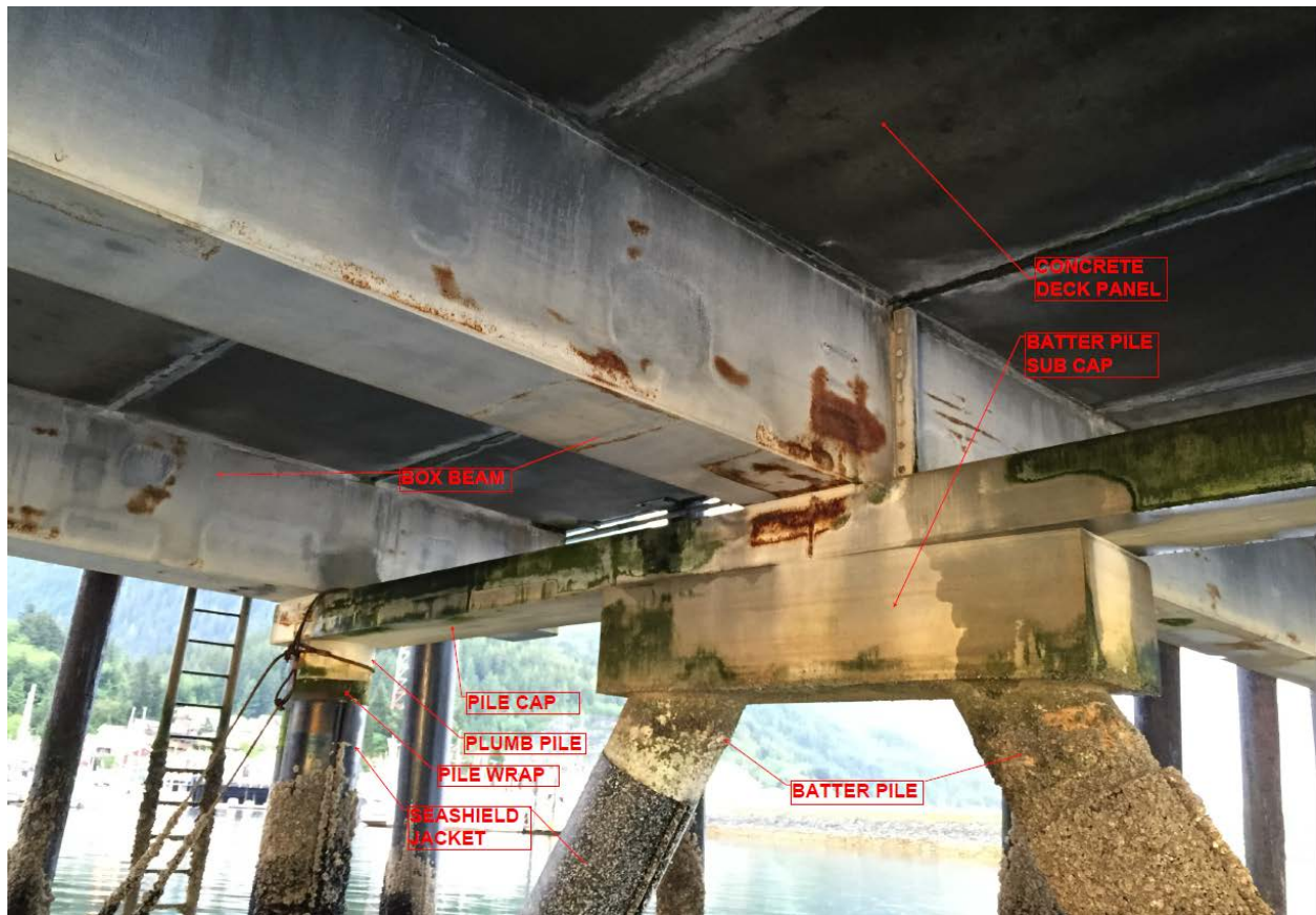
Figure 1.1 - Typical Superstructure
