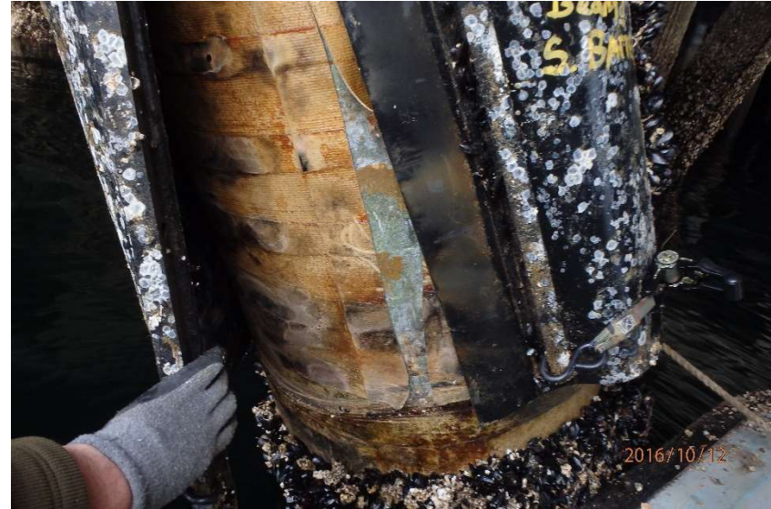
Tape wrap found in good condition
