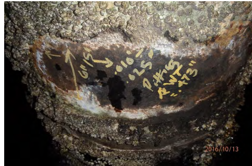
Pile 1, corrosion above pile jacket. (UT Location 1)
