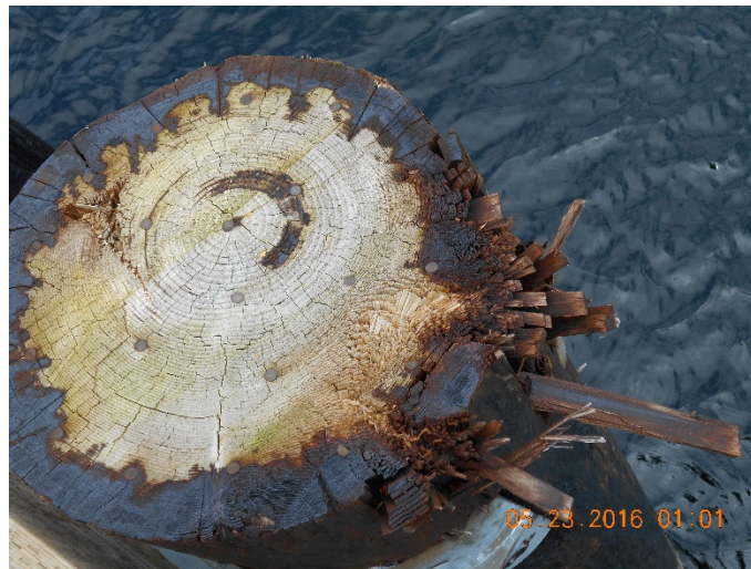
Figure 42: Fender Pile Top With Minor Damage
