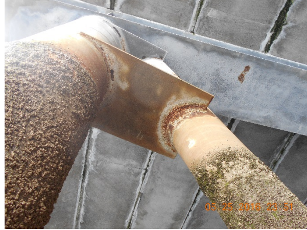
Figure 51: Corrosion at Connection
