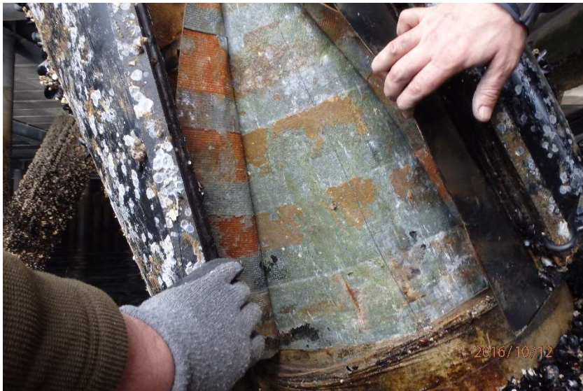
Piling surface beneath tape found in good condition
