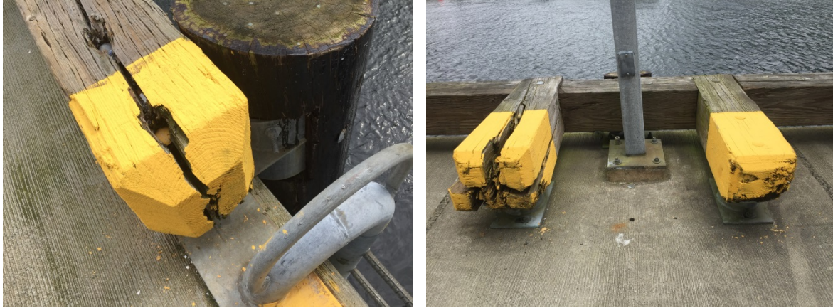
Figure 41: Damaged Bullrail Sections
