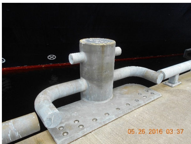
Figure 52: Bollard Abrasion and Corrosion
