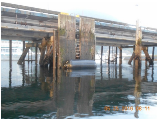
Figure 9a: Typical Fender Panel
