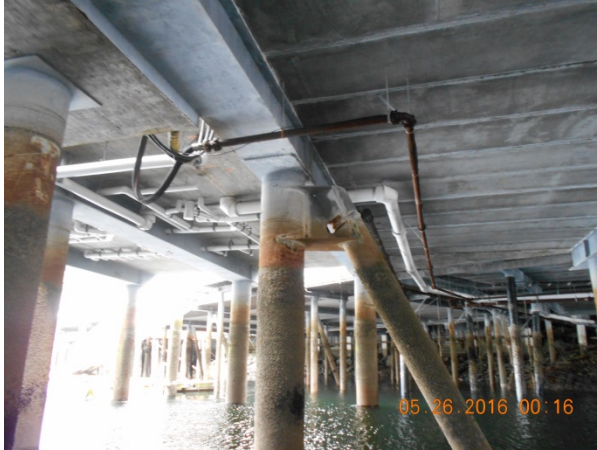
Figure 50: Pile and substructure corrosion
