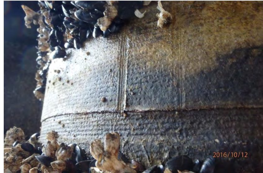
Pile 1, with jacketing gap. Tape wrap intact and not removed.
