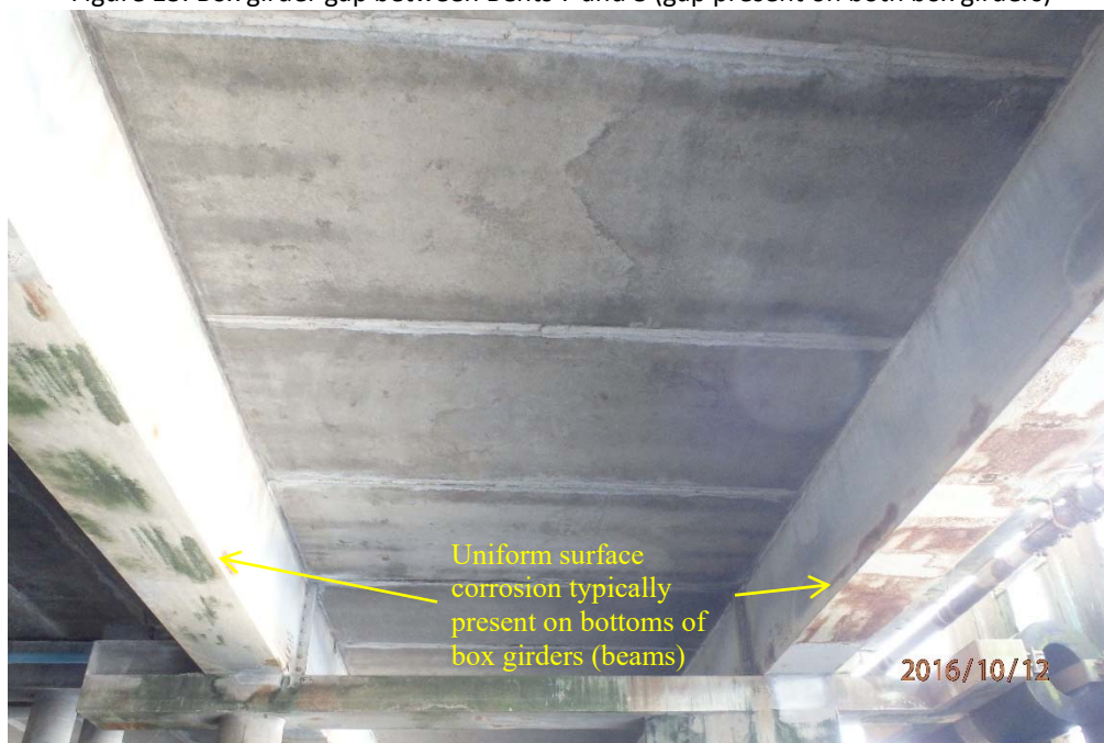
Figure 14: Typical underside of concrete deck panel and girder bottom sides with surface corrosion
