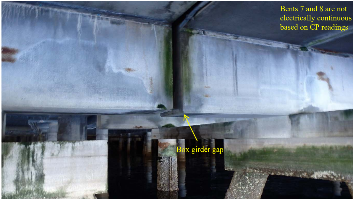
Figure 13: Box girder gap between Bents 7 and 8 (gap present on both box girders)
