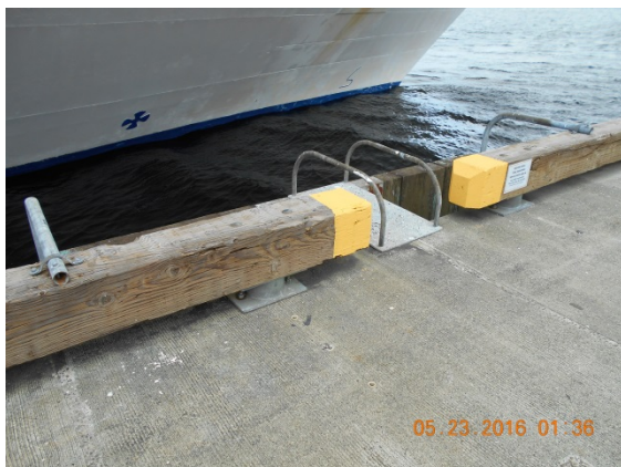
Figure 7: Bullrail and Support
