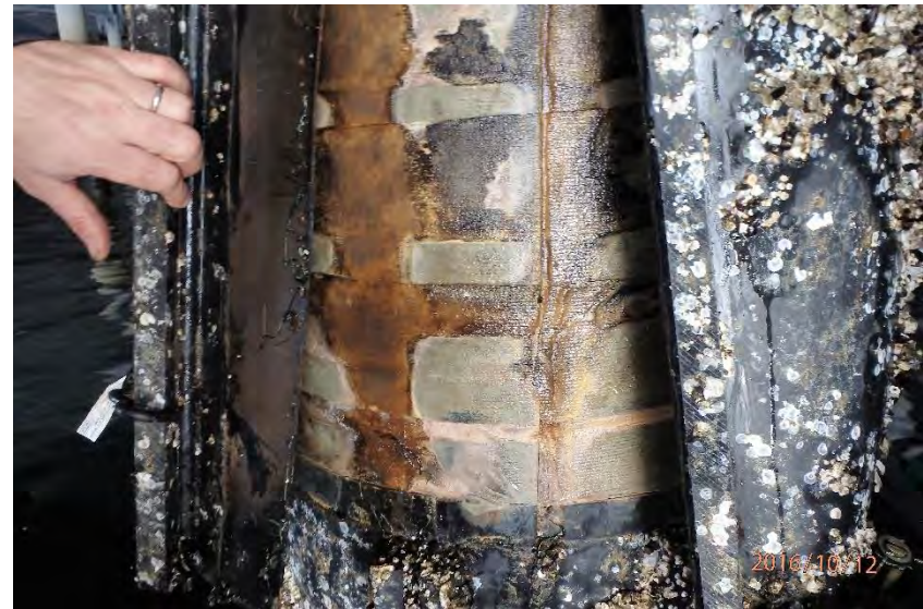
As-found condition of piling tape
