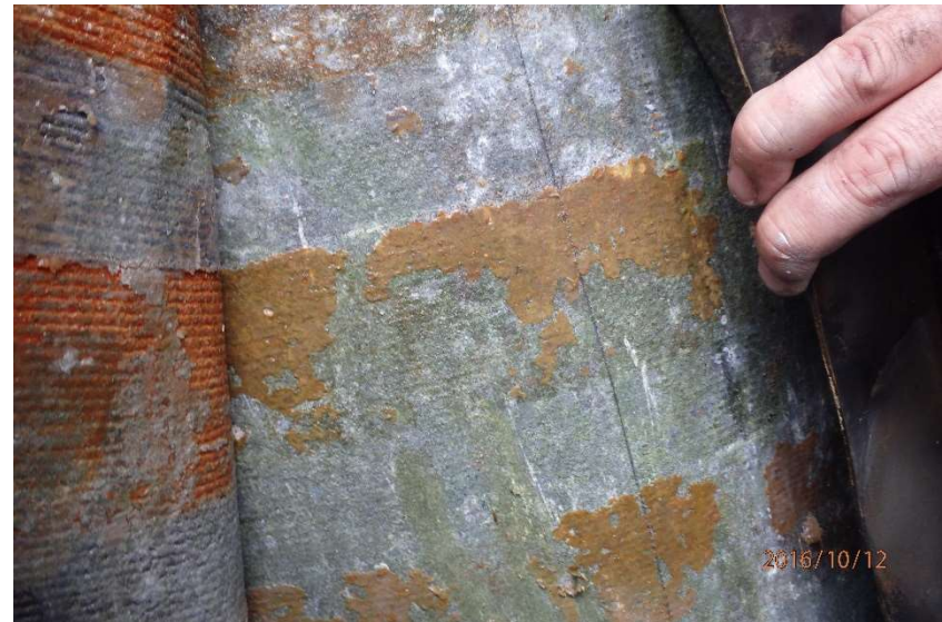
Close-up of piling surface with no visible corrosion
