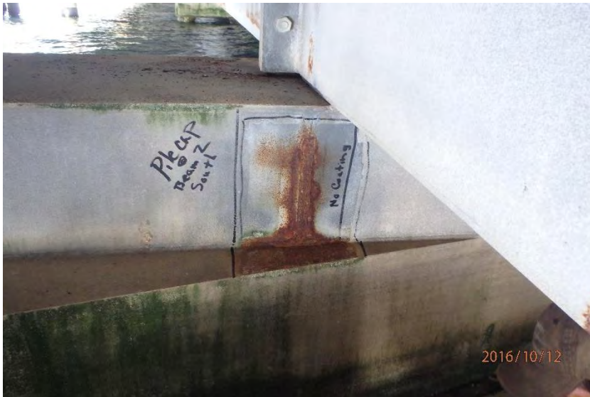
Pile cap weld, south side, under Beam 2 (UT Location 4)
