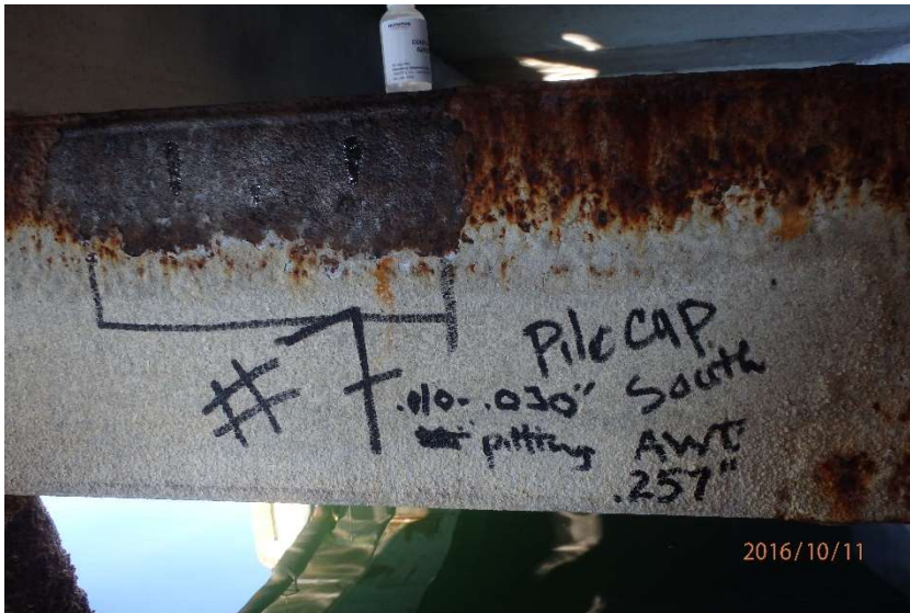
Piling cap, south side (UT Location 1)
