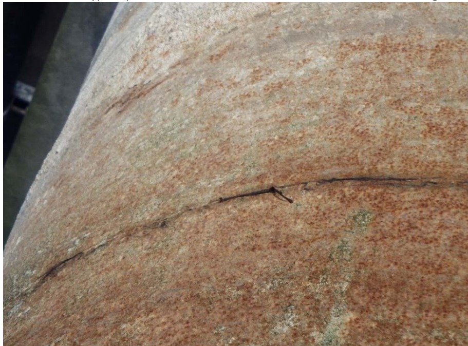
Figure 18: Close-up of typical light surface corrosion on Berth 3 pile
