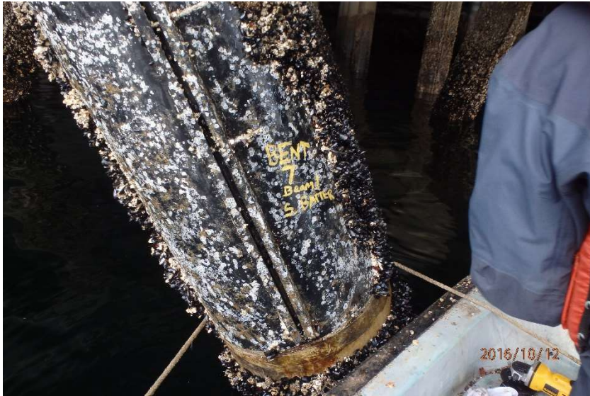
As-found batter pile, south, beneath Beam 1
