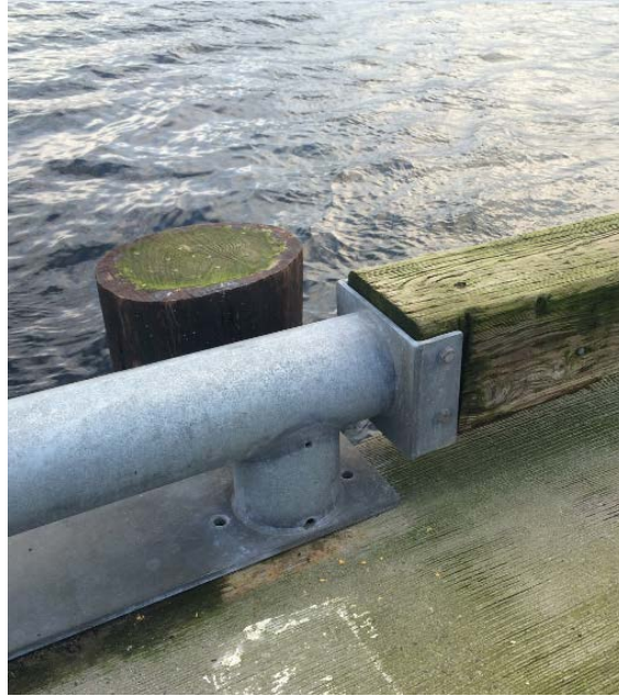
Figure 43: Missing Fender Pile Bolts
