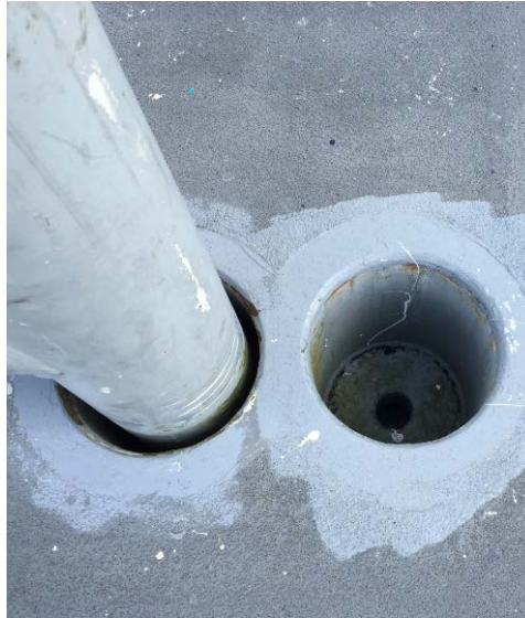
Figure 48: Guard Rail Pockets
