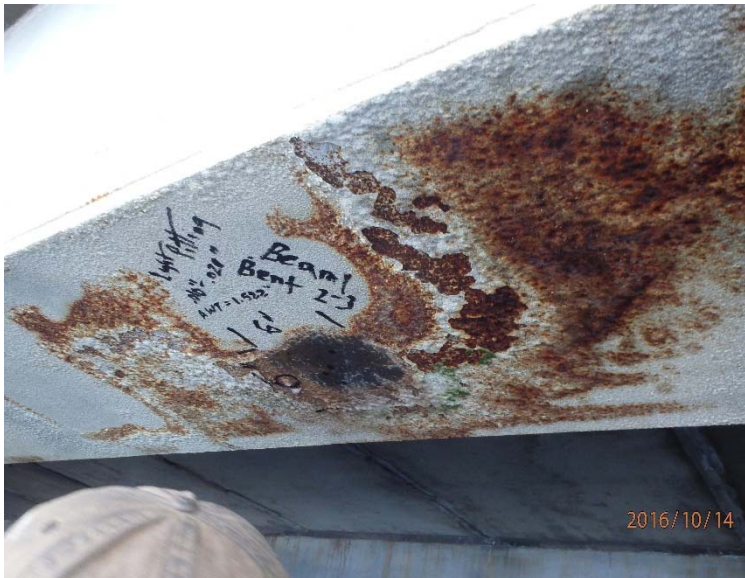
Beam 1 exam area marked with UT and pitting notes
