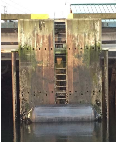
Figure 45: Safety Ladder Blocked by Fender
