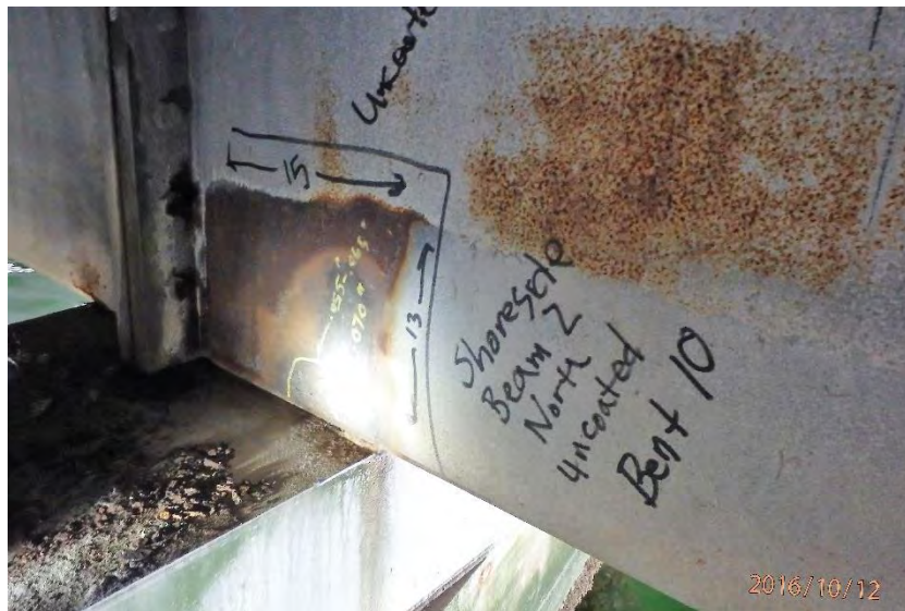
Beam 2 shore side, north end (UT Location 1)
