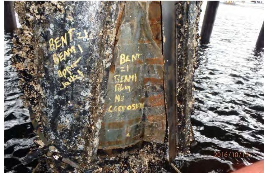
Piling condition at pile sleeve.
