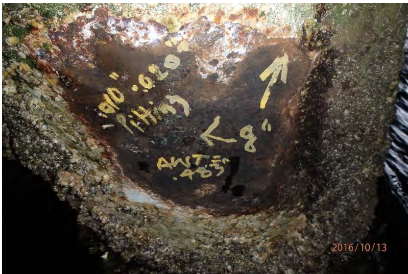
Pile 2, corrosion above pile jacket (UT Location 2)
